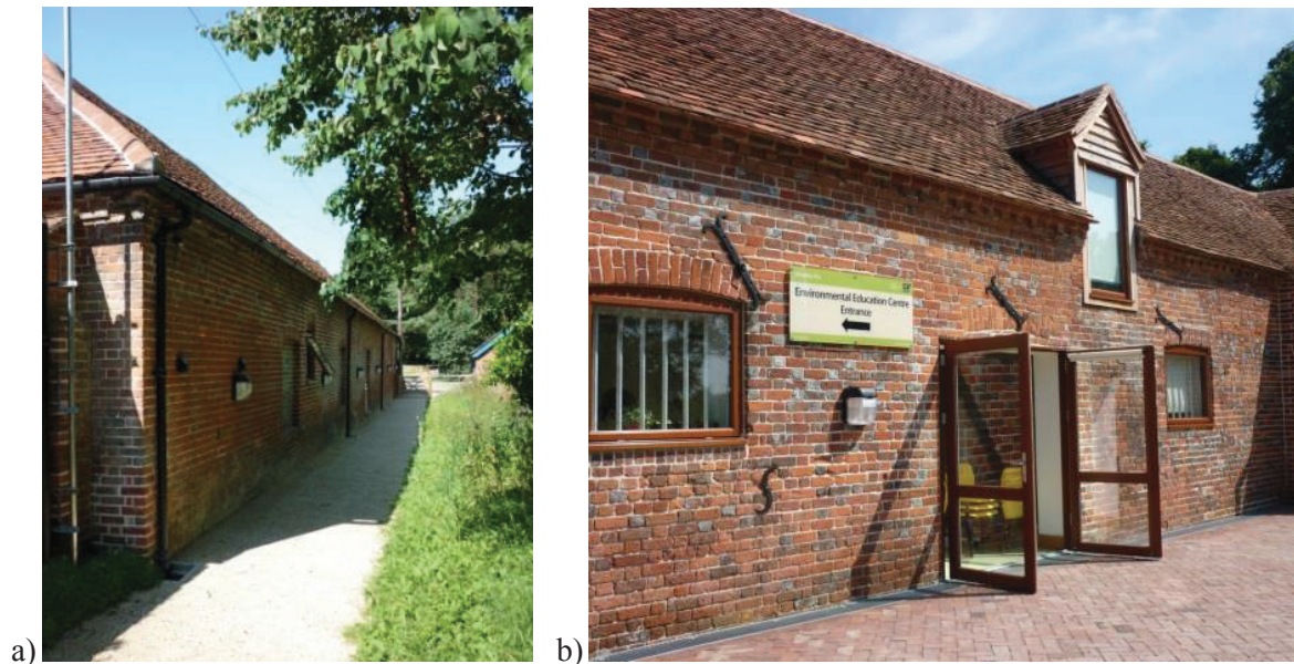
FIG 1. Building and external walls insulated a) north facing wall; b) south facing wall (access to teaching area)
