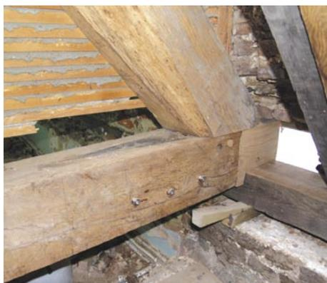
Photo 5: the same beam after repair Repair techniques were devised to maximise the retention of historic fabric and surface finishes so that archaeological evidence, such as carpenters marks could be retained.
